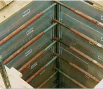
Special solution: manhole lining with additional struts
